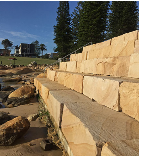
Protection Structure at South West Rocks
